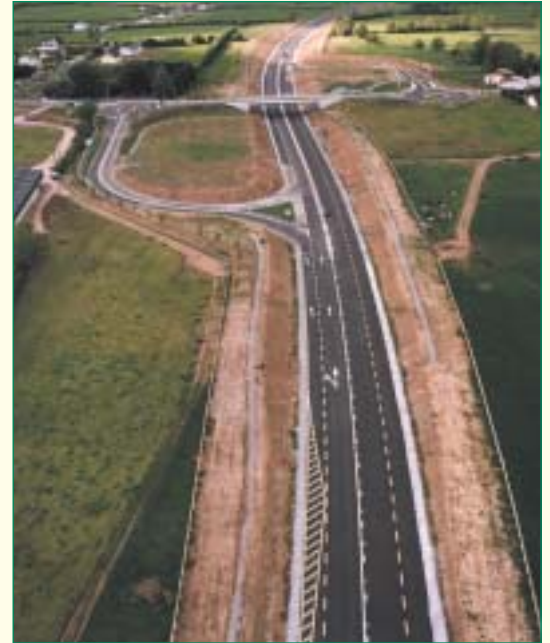
Ballingarry Road Interchange onto N20 Croom Bypass
